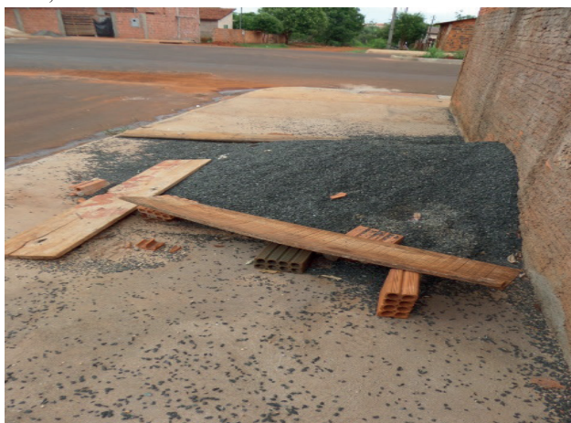
Figure 1 - Construction materials in the path of the residence from S8 to USF. March 2016. Tangará da Serra, Mato Grosso State, Brazil
